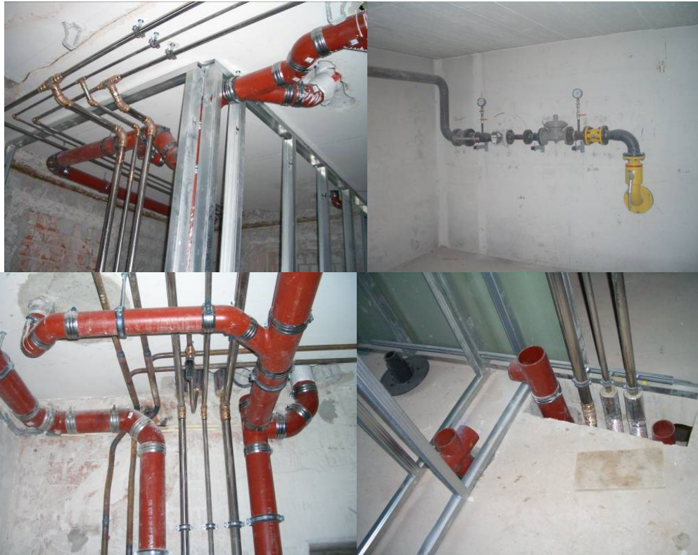
plumbing details during construction
